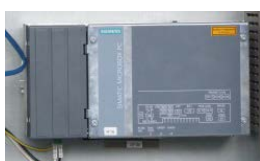
Picture 3-2) Optional industrial computer (IPC, picture shows type EQ2692-...) within large cabinet Type AC-2161 only.
