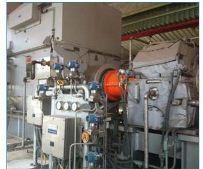
Figure 1. Propylene refrigerant compressor
