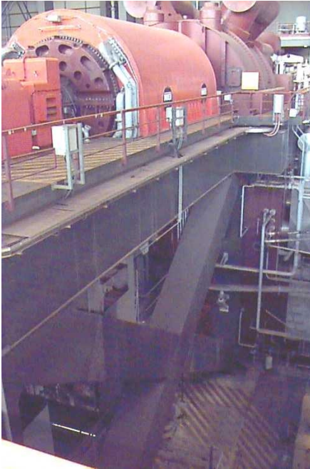
Fig. 2 Flexible steel-beam foundation for earthquake protection
