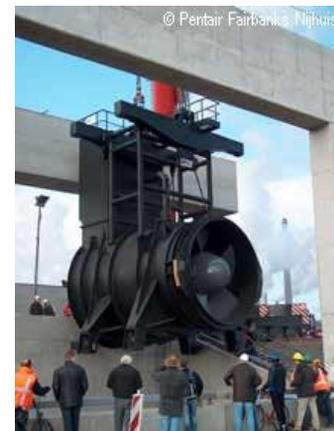
Figure 2. The two new Pentair Fairbanks Nijhuis propeller pumps are type HP1- 4000.340, each with a capacity of 50 m<sup>3</sup>/s and a discharge head of 0.5 to 5 m. Variable speed direct drive 1500 kW motor with 80 RPM maximum speed
