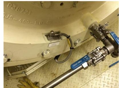
Figure 4. Sensor type and location for the Pentair Fairbanks Nijhuis propeller pump.
