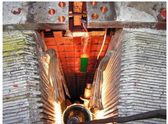
Figure 3. Mounting of the air gap sensor (green plate) and the magnetic flux sensor (right) between two poles on the stator laminates.
