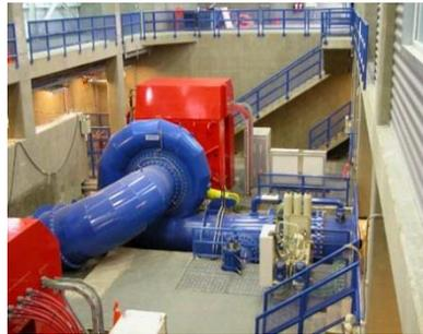
Figure 2. Typical Andritz Hydro compact hydrogenerating unit (horizontal Francis turbine, 9.2 MW).
