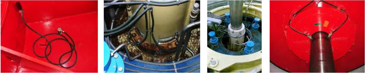
Figure 4. Examples showing sensor installation on the hydro generating units. On the far left is the velocity sensor on the generator top cover for monitoring axial vibrations. The two photos in the middle show the X-Y radial displacement sensors mounted just over the turbine guide bearing. On the far right are the X-Y radial displacement sensors mounted below the lower generator guide bearing.
