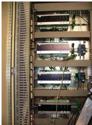
Figure 5. Typical cabinet installation for the compact monitors.
