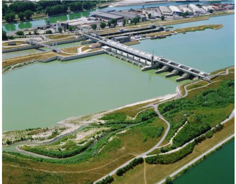
Figure 2. Freudenau hydroelectric power station.
