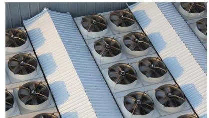
Figure 1. Induced draft air coolers
