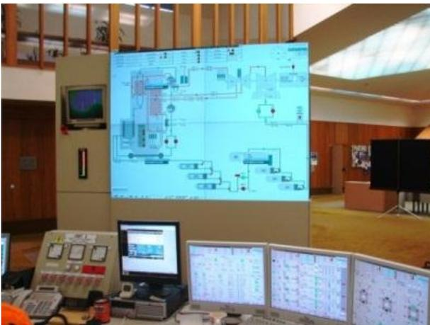
Figure 10 Analogue control and DCS for one Unit
