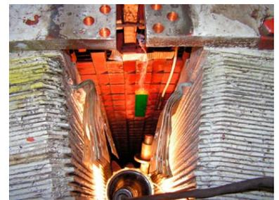
Figure 2. Mounting of the air gap sensor (green plate) and the magnetic flux sensor to the right of the air gap sensor between two poles on the stator laminates.
