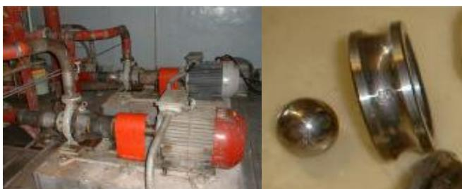
Figure 10. There are three demineralized contaminated water pumps for each reactor unit. Each 55 kW motor-driven pump has a flow capacity of 90 m<sup>3</sup>/hr at 3000 rpm. Damaged bearings are shown in the picture to the left.
