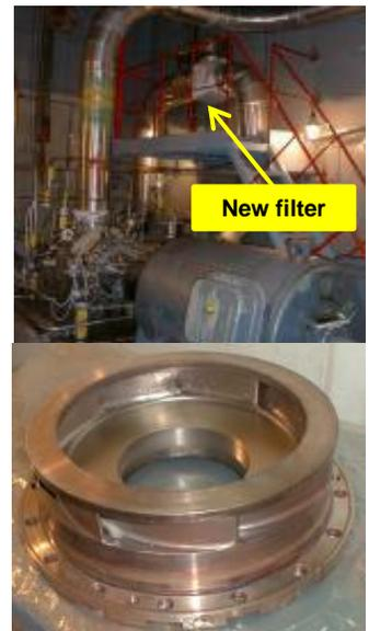
Figure 8. There are two purification and cooling system pumps for each reactor unit. Each 500-kW motor-driven pump has a flow capacity of 500 m<sup>3</sup>/hr at 3000 rpm. A damaged shroud is shown to the below.
