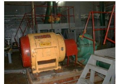
Figure 5. There are six accident confinement pumps for each reactor unit in the condenser tray cooling system. Each 320-kW motor-driven pump has a flow capacity of 1250 m<sup>3</sup>/hr at 1500 rpm.
